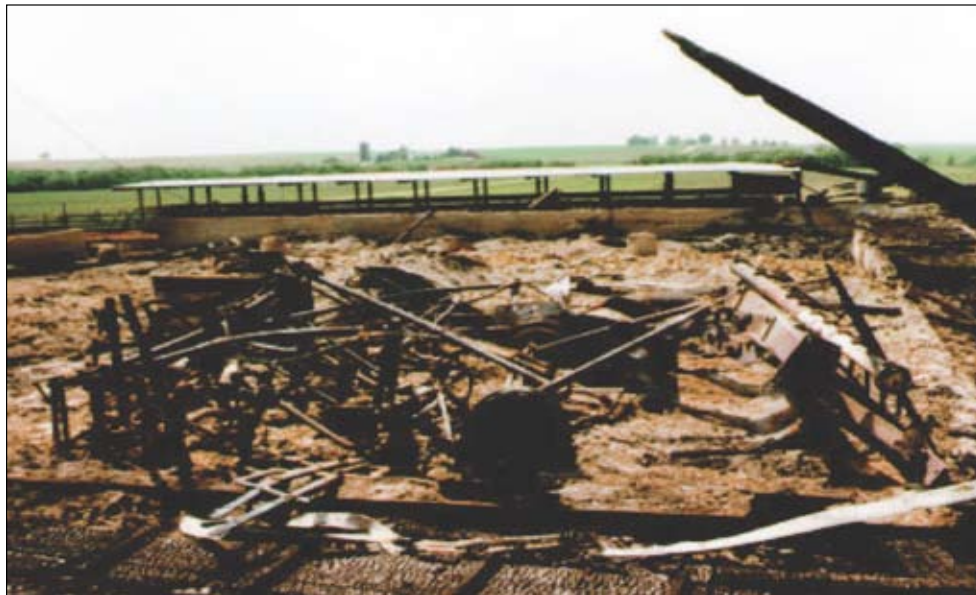
Destruction of farm buildings due to extension of spontaneous combustion-caused fire in silo
