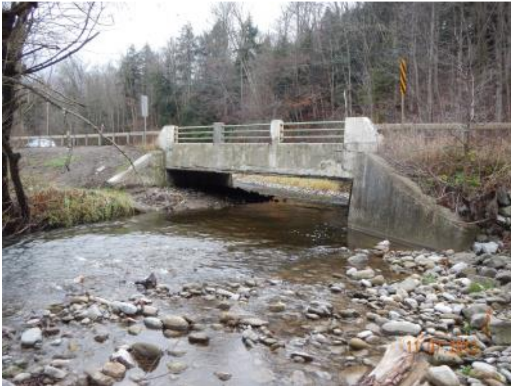
Photo Source: Milone & MacBroom, Inc. (2013)
