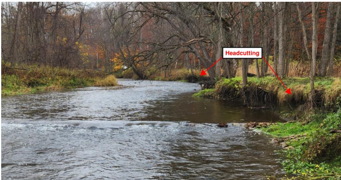
Figure 8-30. Headcutting upstream of Lombard Road at RS 742+00.
