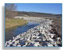
To prevent future erosion on a river bend, incorporate rock vanes to deflect current away from the bank.
