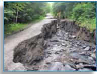
After severe flooding, an undamaged stream reach comparable to a damaged section may be difficult to find. In these circumstances, stream-channel dimensions can be calculated using the Bank-full Hydraulic Geometry Tables for Selected Hydrologic Regions (Regional Tables). Find directions for using Regional Tables on DEC's website at www.dec.ny.gov/lands/86450.html
