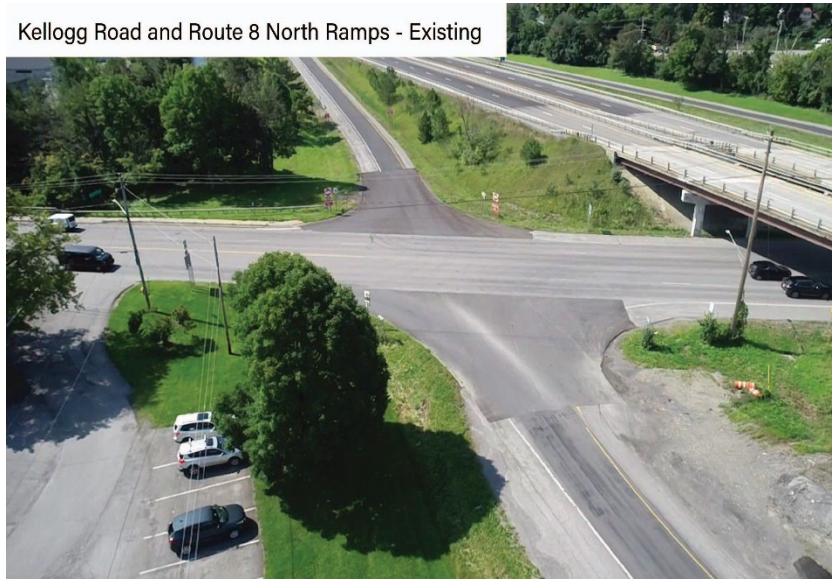
Kellogg Road and Route 8 North Ramps
