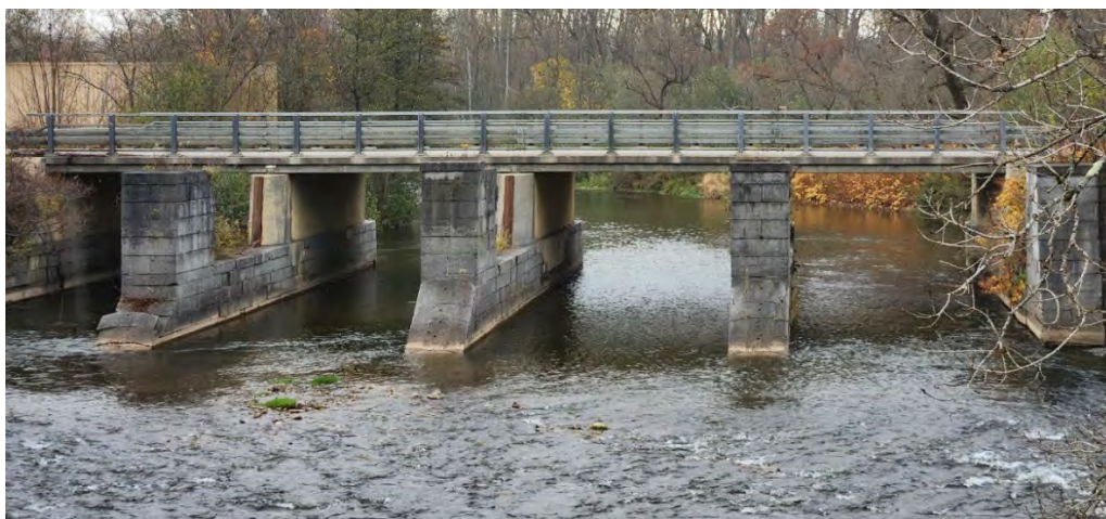
Figure 8-39. In-channel piers at NY-69/Erie Boulevard in the Town of Whitestown, NY.
