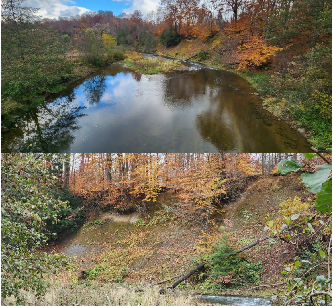
Figure 8-32. Bank erosion downstream of Valley Road, Town of Whitestown, NY.
