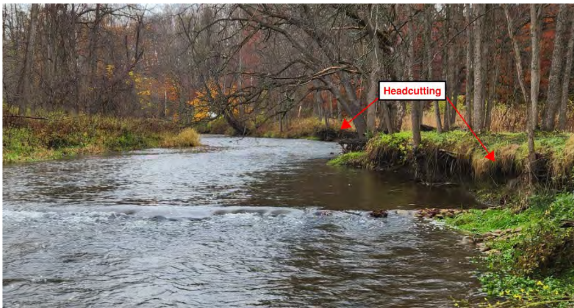
Figure 8-30. Headcutting upstream of Lombard Road at RS 742+00.
