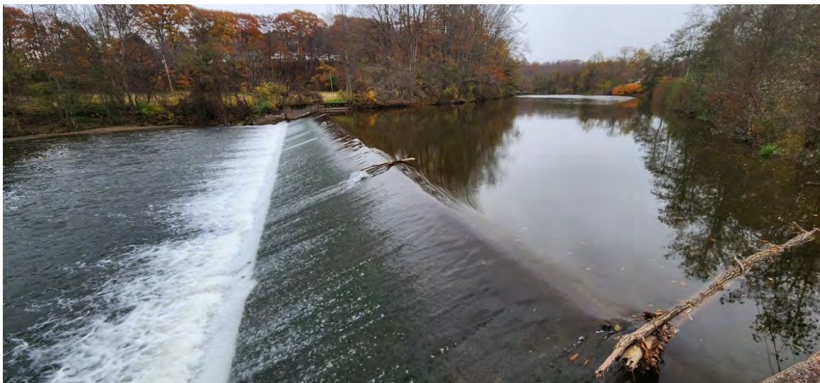
Figure 8-34. Oriskany Falls Dam in the Town of Whitestown, NY.
