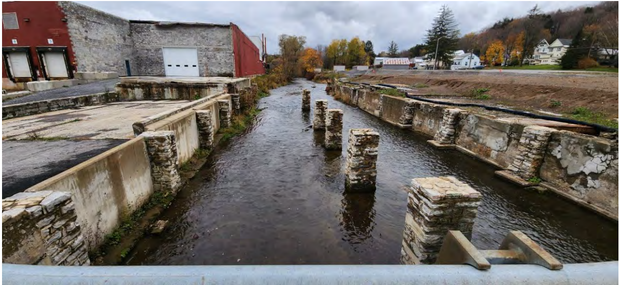
Figure 8-7. In-channel piers upstream of Division Street in Oriskany Creek.
