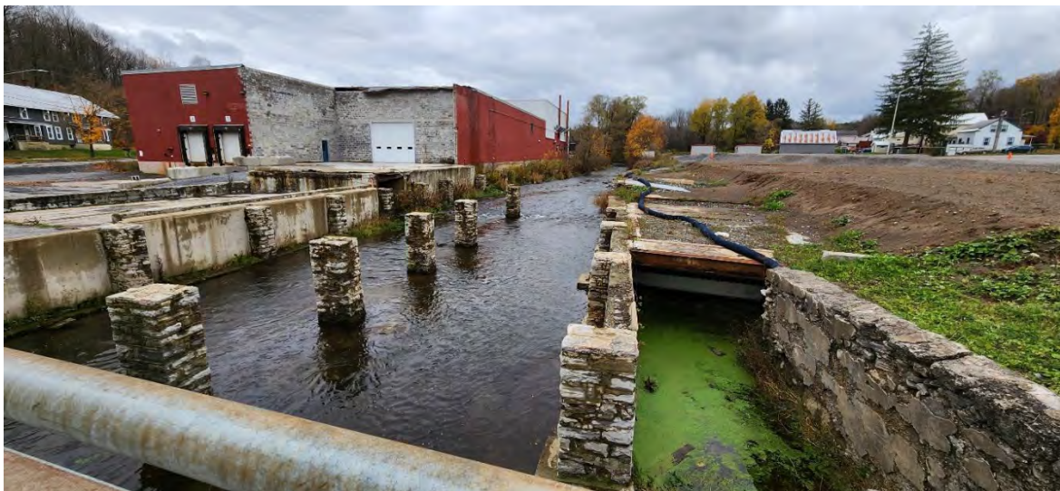
Figure 8-12. Current conditions of the property looking upstream of Division Street.
