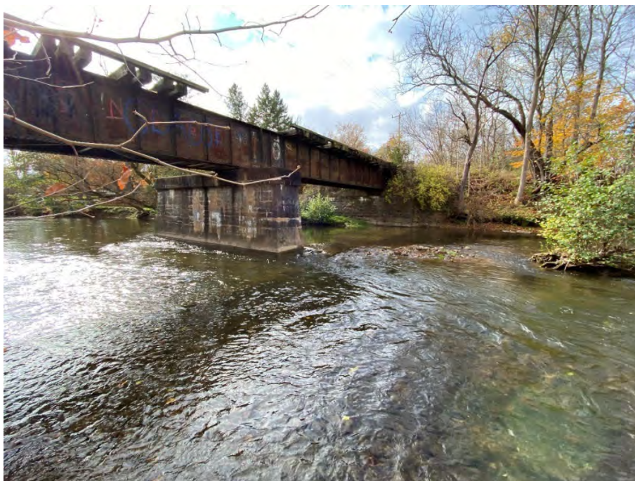
Figure 8-28. Existing conditions of the abandoned railroad bridge in Village of Clarks Mills, Kirkland, NY.
