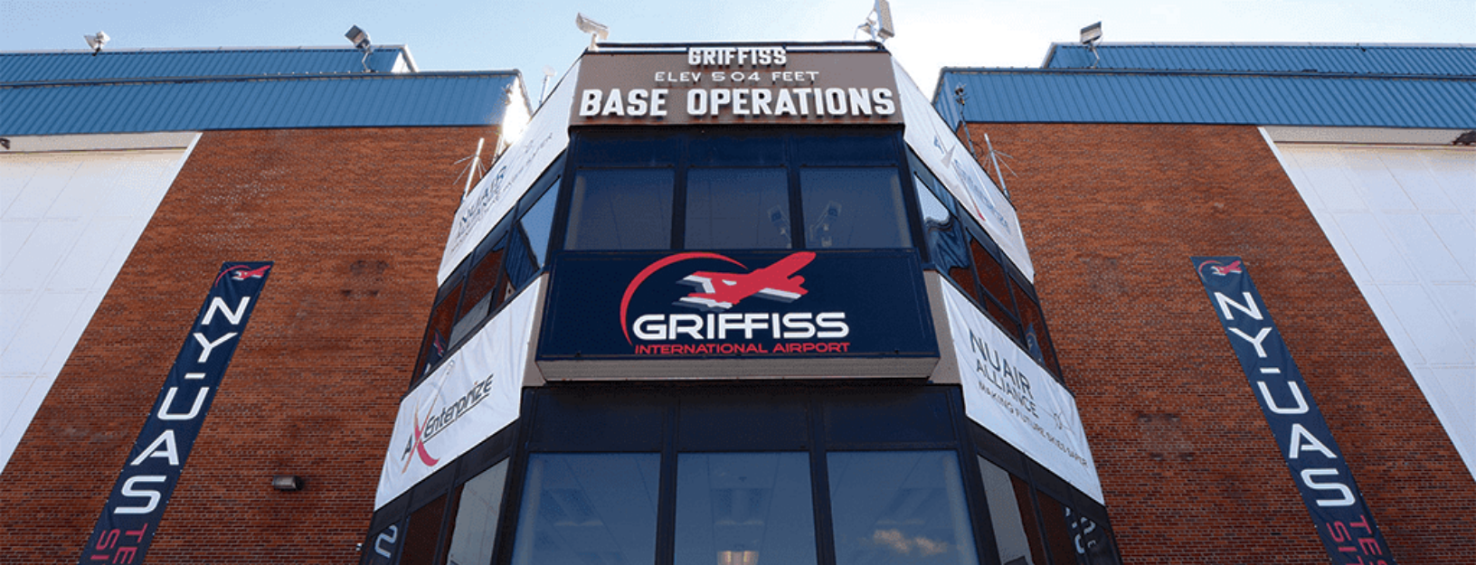
FIGURE 5.5: NY Unmanned Aerial System Test Site, at Griffiss International Airport
