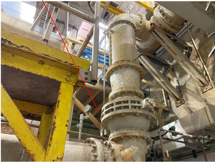
Photo 9 – Valve CV-0021: 16" Ball valve. Representative of valves CV-0022, CV-0023, and CV-0024. All four to be replaced in future project
