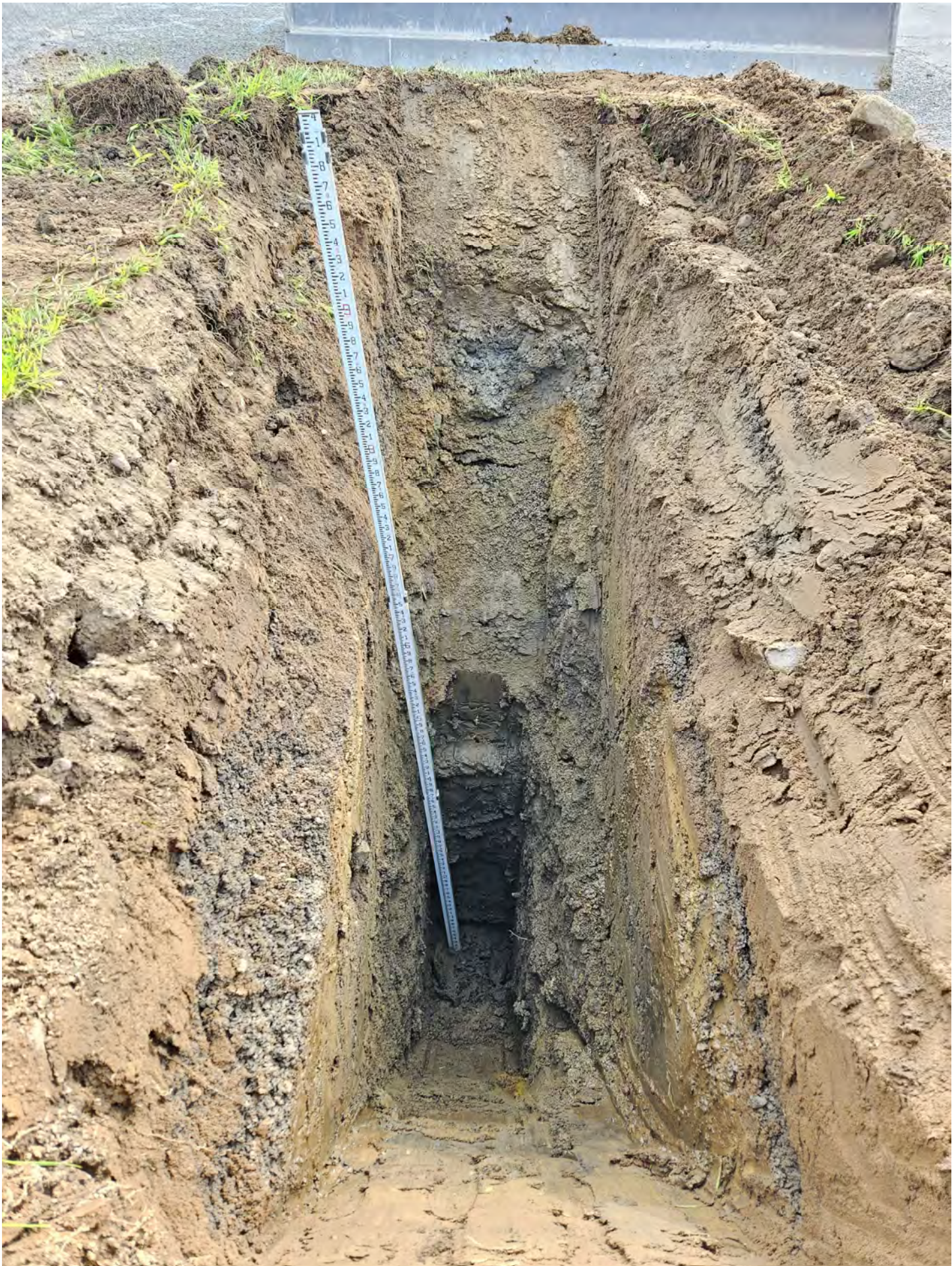
Photograph 5: Test Pit TP-6
