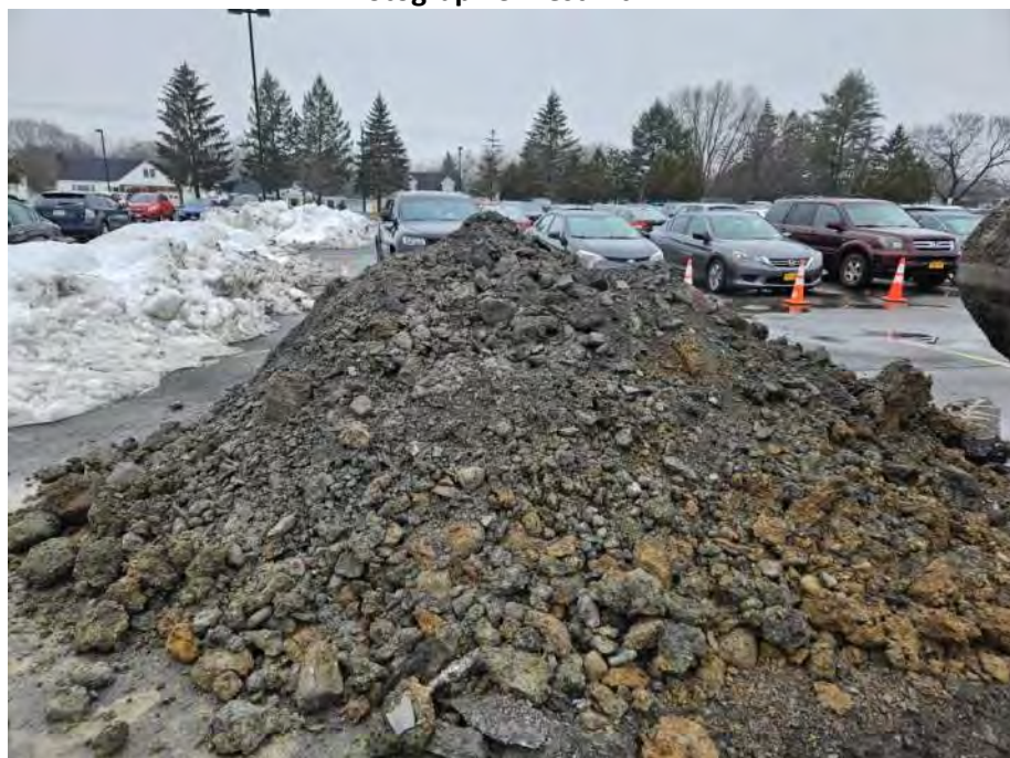
Photograph 4: Test Pit TP-2
