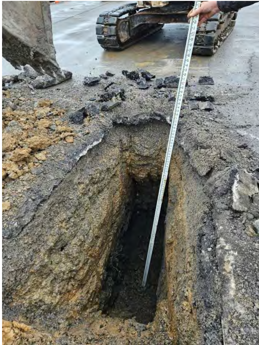
Photograph 3: Test Pit TP-2
