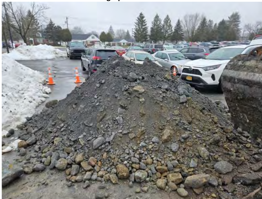
Photograph 6: Test Pit TP-3
