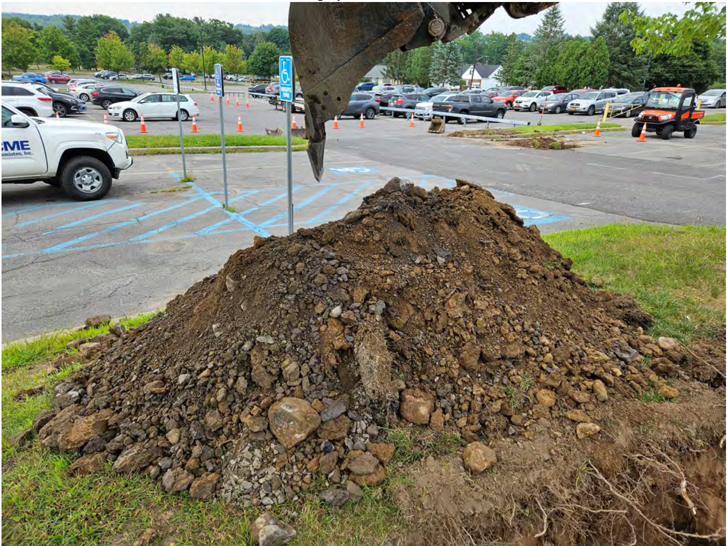
Photograph 4: Excavated Material From Test Pit TP-5
