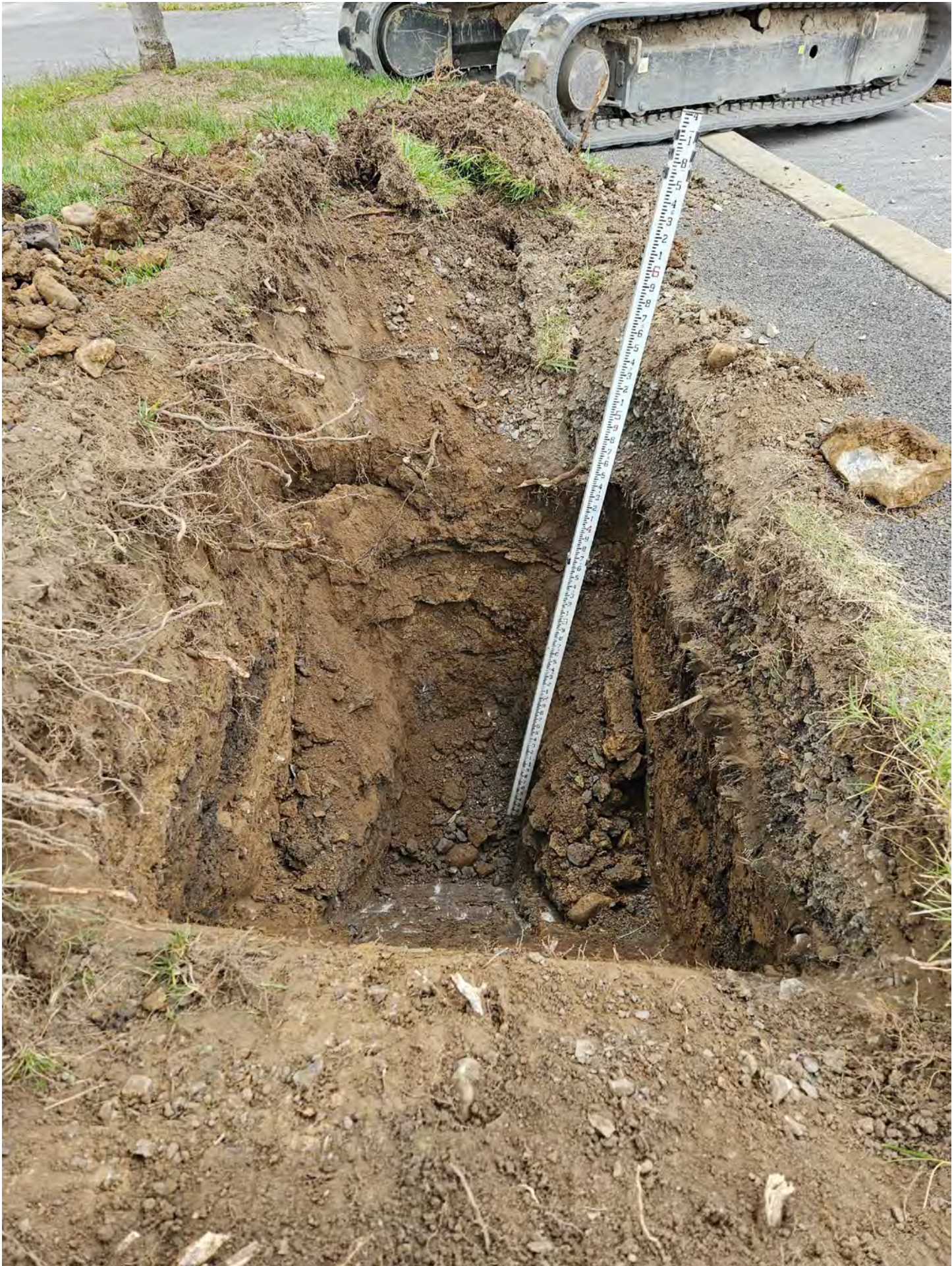
Photograph 3: Test Pit TP-5
