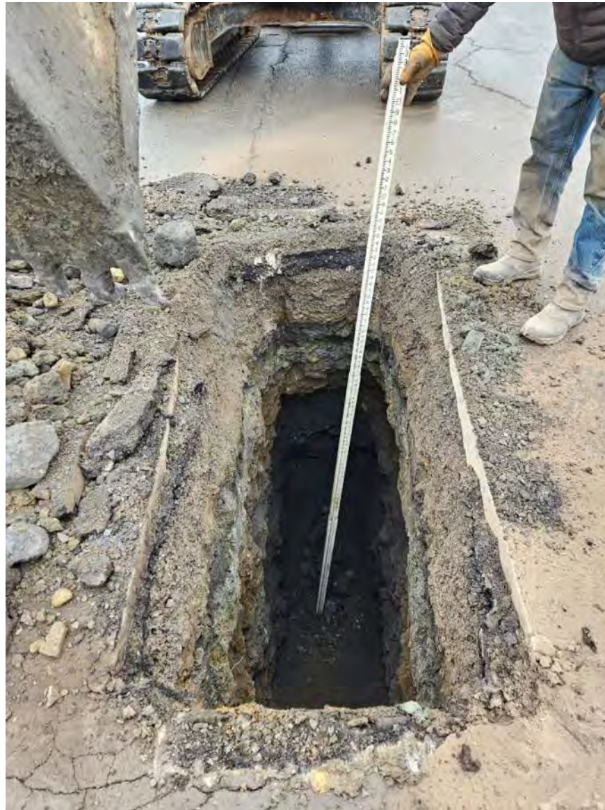
Photograph 5: Test Pit TP-3
