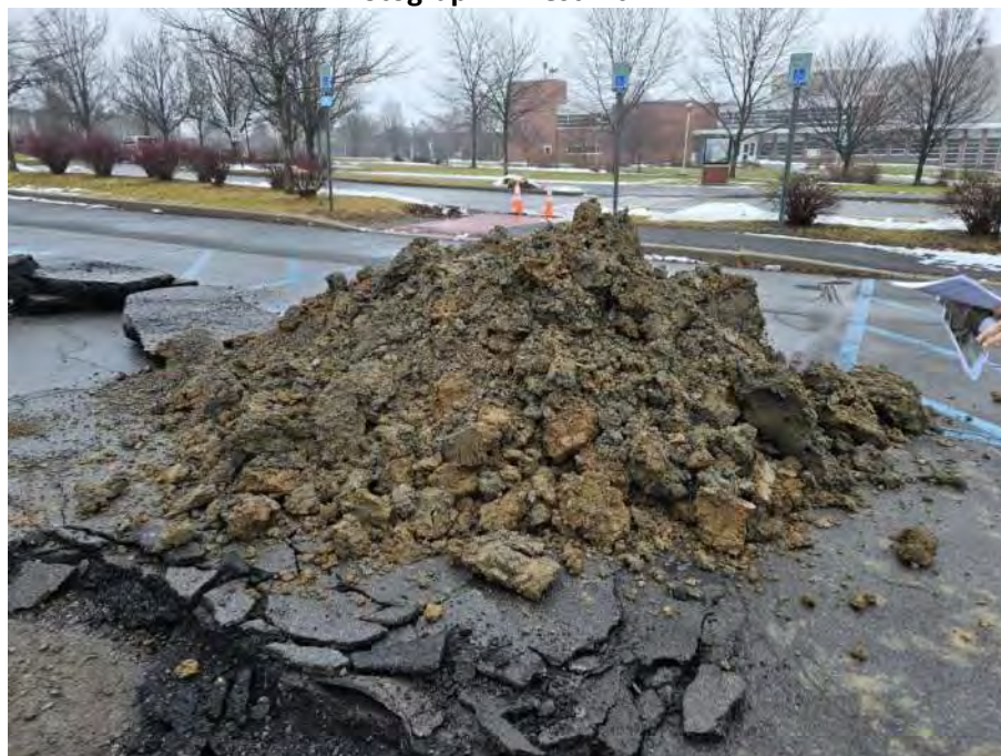
Photograph 2: Test Pit TP-1
