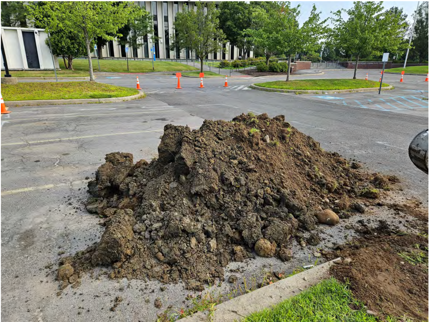
Photograph 6: Excavated Material From Test Pit TP-6
