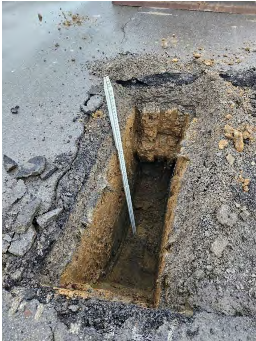
Photograph 1: Test Pit TP-1
