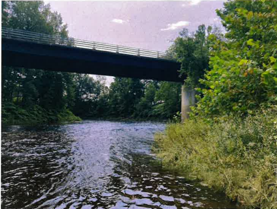
PHOTO A - View facing downstream of the Oswego Road Bridge.
